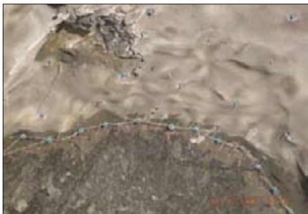
Figure 11. Example of "hanging up" spiling at the Bærums tunnel, photo National Rail Administration.
