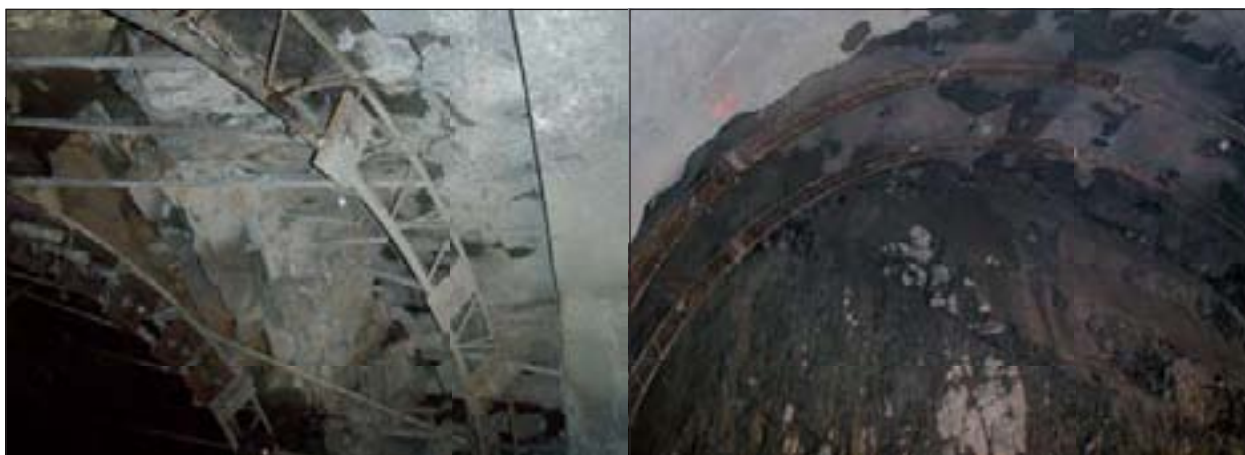
Figure 16 Example of the use of lattice girders from the construction of a subway (T-baneringen in Oslo)
