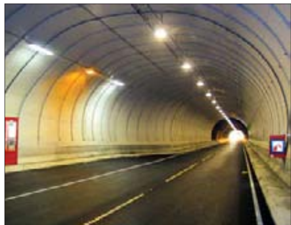
Installation of WG Tunnel Arch in the Rotsethorntunnel, Norway.
