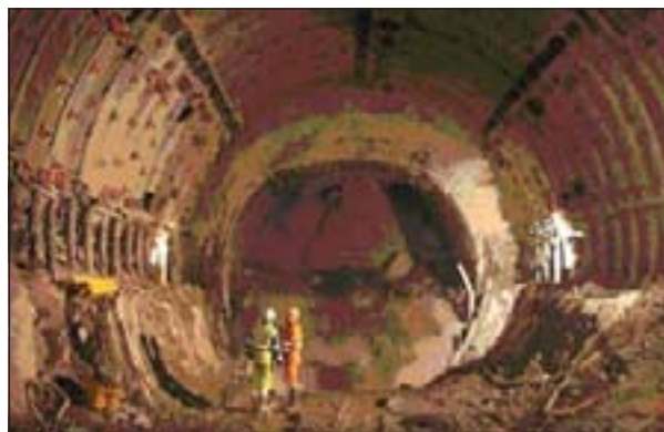
Figure 17. Deformable support system for high rock stress and big deformation. From the new St Gotthard railway tunnel, photo Amberg Engineering.
