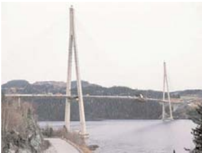
The Skarnsundet Bridge is a 1,010 m long cable stayed bridge with 12 spans. The main span is 530 m long and the A-towers are 152 m high. Veidekke was honoured by the National Association of Architects for this project.
