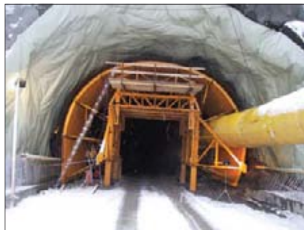
Figure 19. The picture shows an example of the Flexi form that was used at the access tunnel to Melkøya
