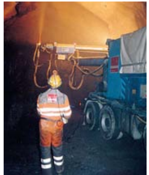
A shotcrete robot working its way through the Norwegian mountains.
