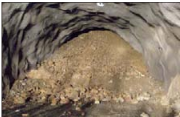
Figure 46: Face collapse. The picture was taken the day after the start of the collapse
