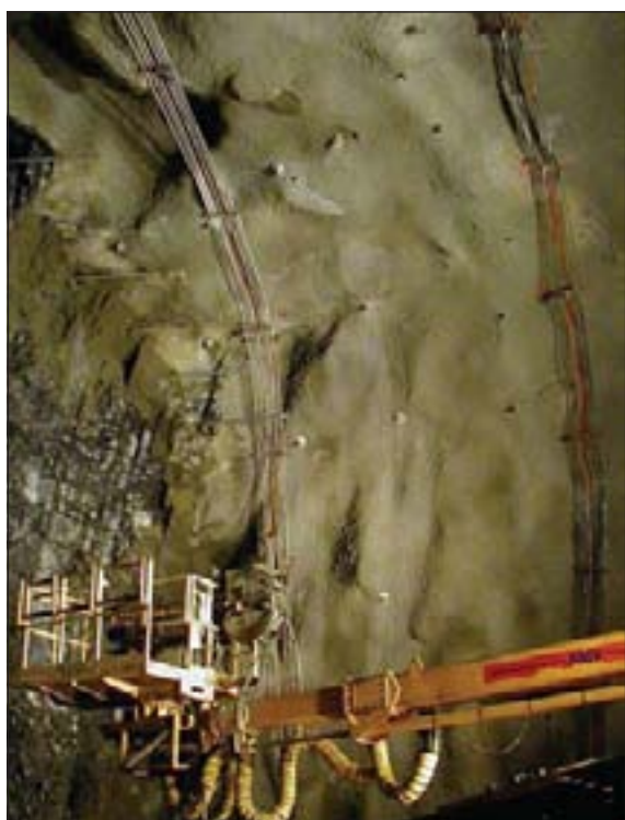
Figure 14. Reinforced sprayed concrete ribs from the Tanum tunnel and at the National Theatre Station respectively
