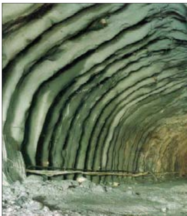
Figure 14. Reinforced sprayed concrete ribs from the Tanum tunnel and at the National Theatre Station respectively
