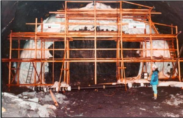
Figure 6.7. Ground freezing in the Festnings tunnel
