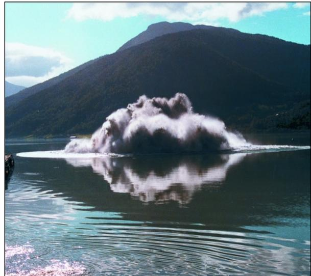
Figure 3.5. Piercing of the tailrace tunnel for Jostedal hydropower plant at 40m depth in Gaupnefjorden (Statkraft)
