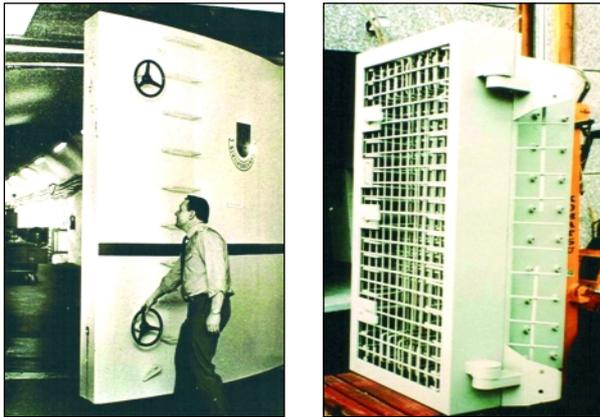
Figure 3.14. Typical blast gate and blast door
