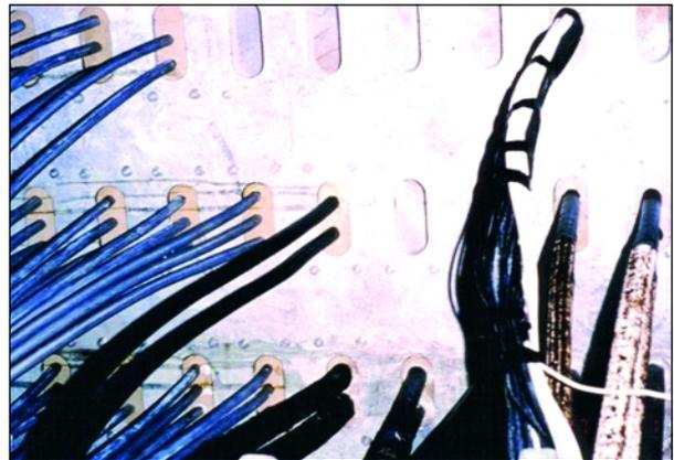
Figure 3.13. Cables entering the blast barrier
