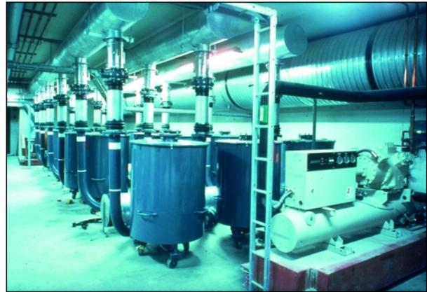
Figure 3.15. Gas filters in an underground facility
