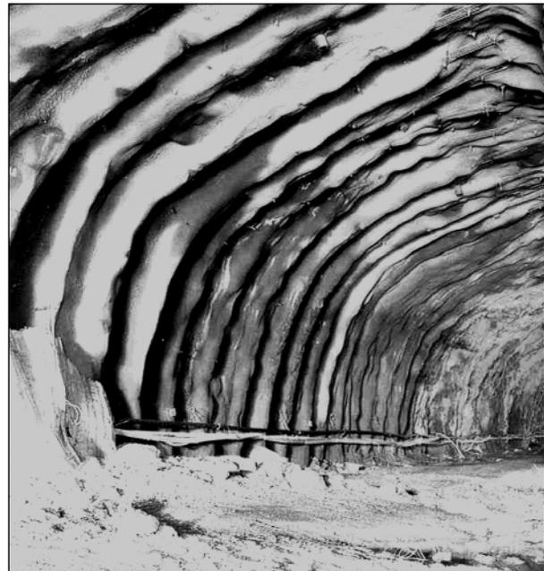
Figure 6.3. Reinforced ribs of sprayed concrete at Nationaltheateret railway station
