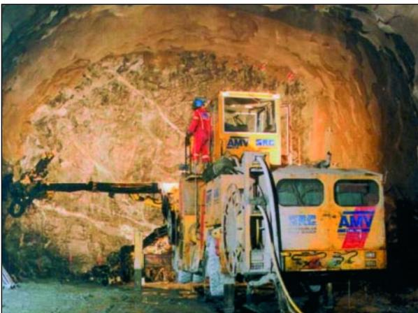
Figure 7.1. Modern drilling jumbos
