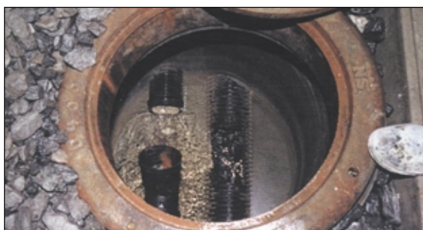
Figure 4. Permanent side drain entering the main drain (NSB Gardermobanen).
