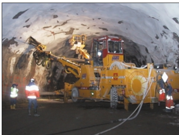
Baneheiea. Drilling of grout holes.
