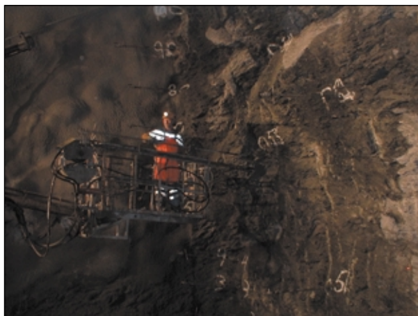
Fig. 2. Grouting works in the Storhaug tunnel
