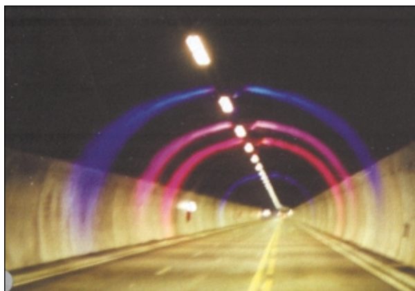
Fig. 1. The completed Oslofjord tunnel with artistic light effects for driver's comfort. No water seepage visible due to cost-effective pre-grouting and water shielding.
