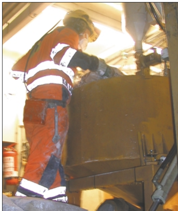
CONTROL OF GROUT MIX.
