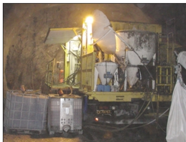
Fig. 1. Grouting equipment in the Metro ring tunnel (photo: Knut Boge)
