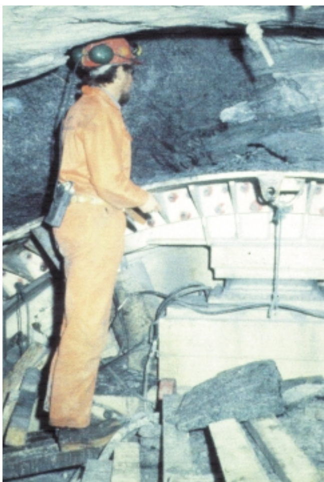
Fig. 4 Rock spalling overbreak in roof
