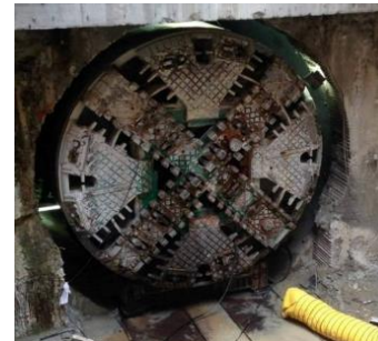
February 2014 Tunnel Breakthrough – Bukit Panjang Bound
