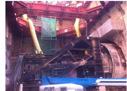
March 2014 Expo Line Launching
