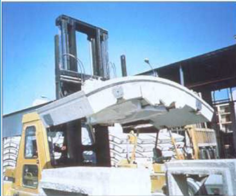
Transportation of precast segments (Metrosud).
