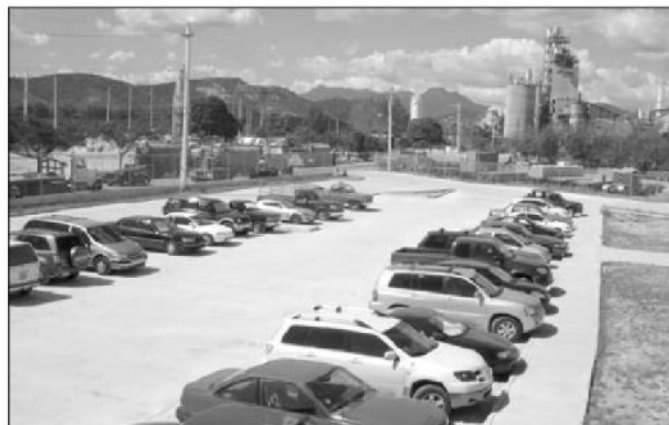
Photo 6.2 - Example of use in the parking areas.
