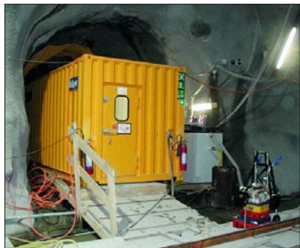
Figure 12.3: Rescue container with oxygen shall be placed maximum 500 m from face.
