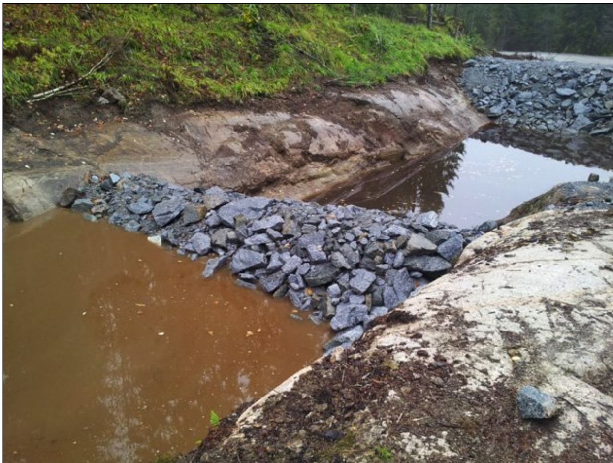
Figure 1 A double camber semi permeable sedimentation pond
