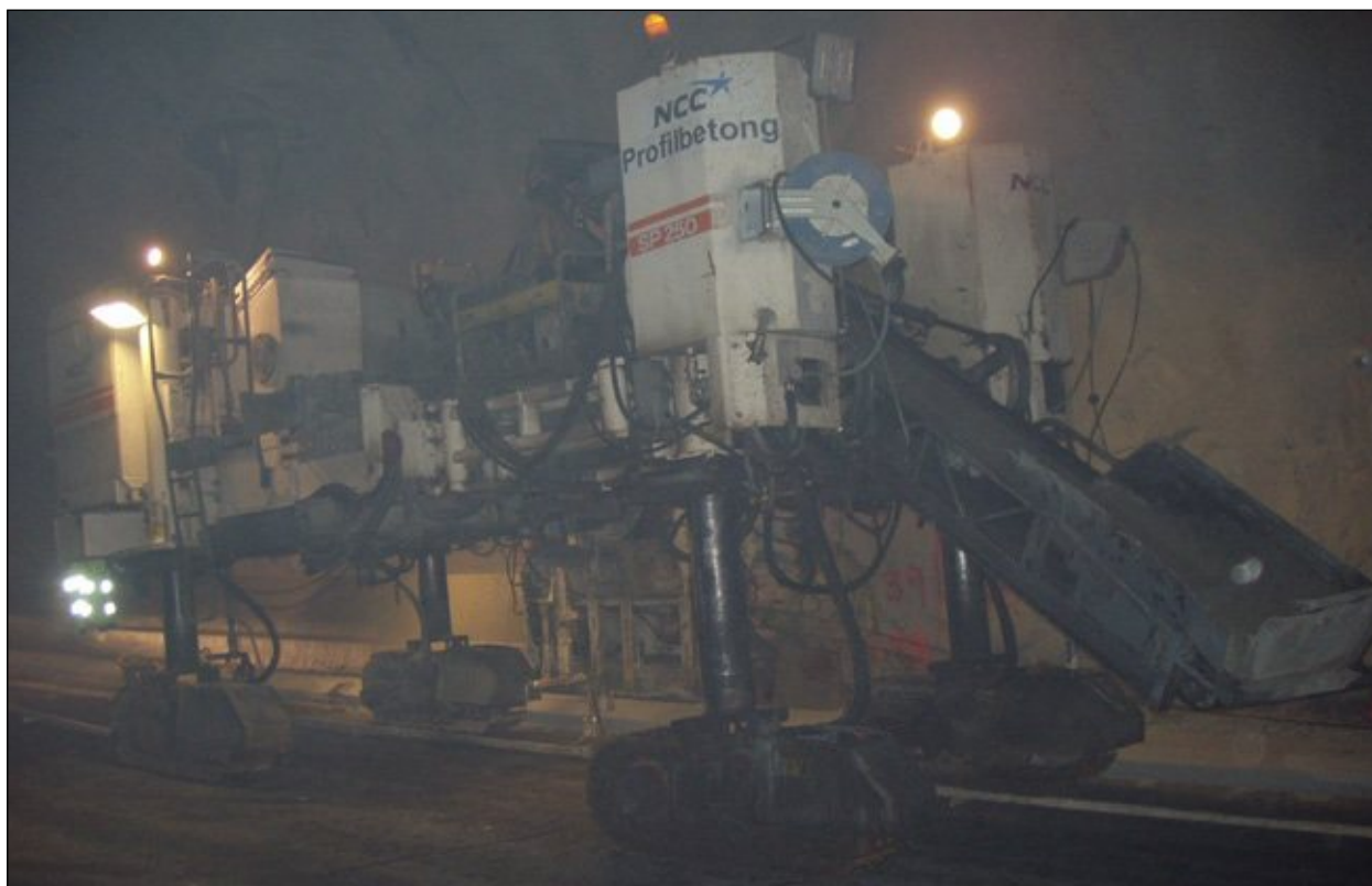
Figure 1: Concrete pouring of barriers
