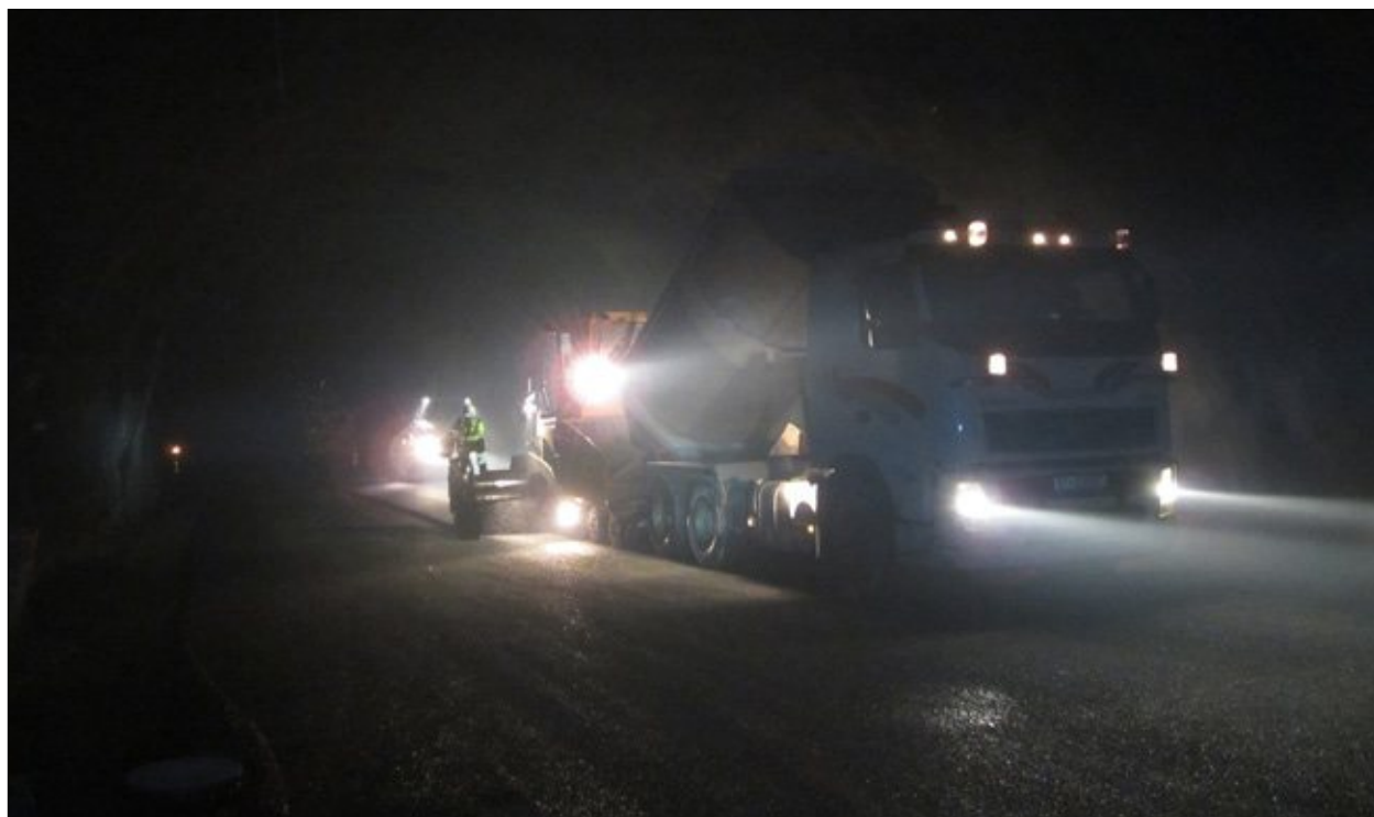
Figure 2: Laying asphalt
