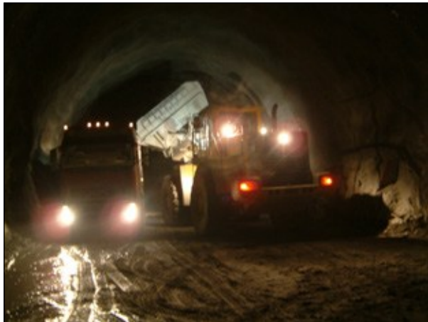
Figure 3: Loading at the face without generating dust
