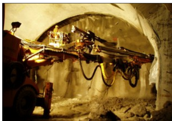
Figure 5. Excavation through the cave-in zone at the Atlantic Ocean tunnel. Pre-grouting was done for coping with large water inflow, and the tunnel face reinforced with sprayed concrete, rock bolts and steel straps for ensuring stability and allowing for high grout pressure.
