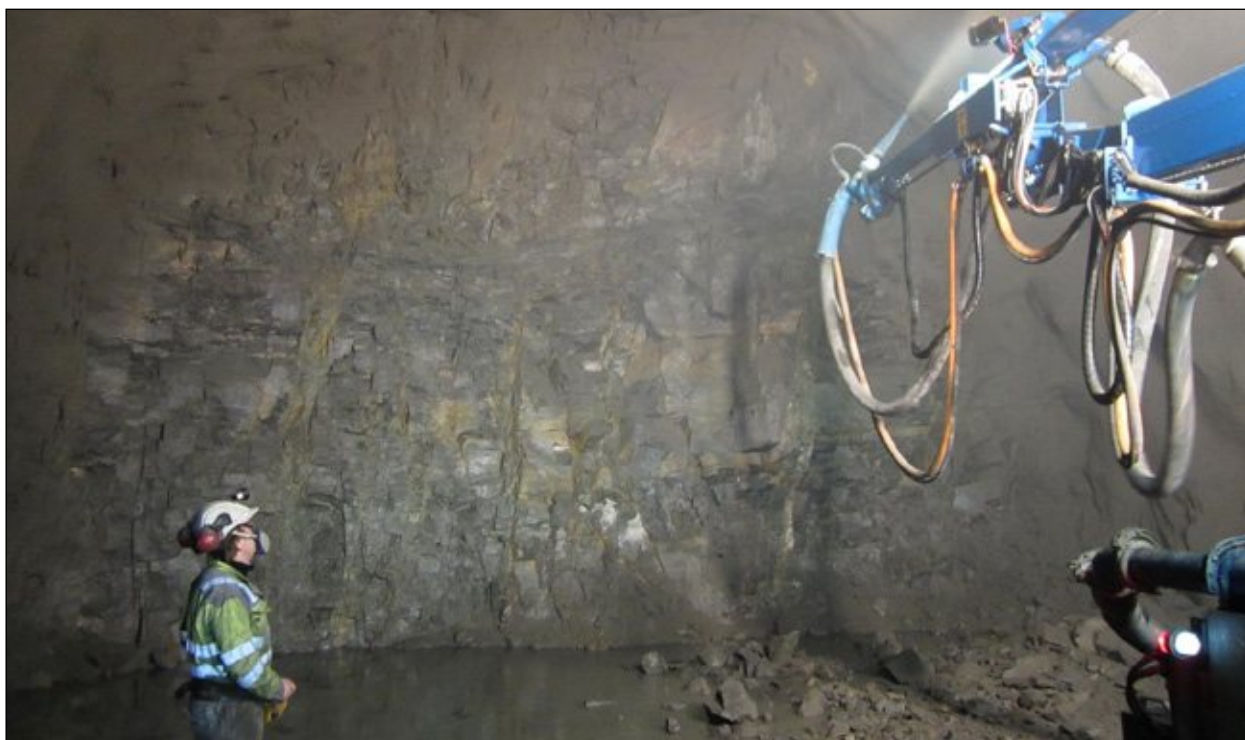
Figure 5: Spraying robot operated by remote control
