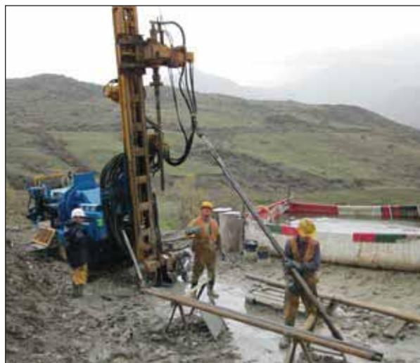
Figure 5: Core drilling in the Flysch
