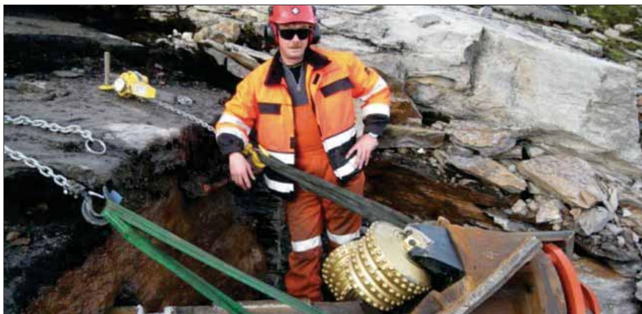
Figure 5. Raise drilling. Ready for reaming the shaft
