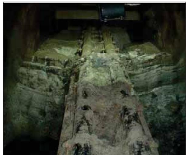
Figure 5: Inspection of the tunnel sand trap after 8 years of operation, from the tunnel sand trap in 2000.
