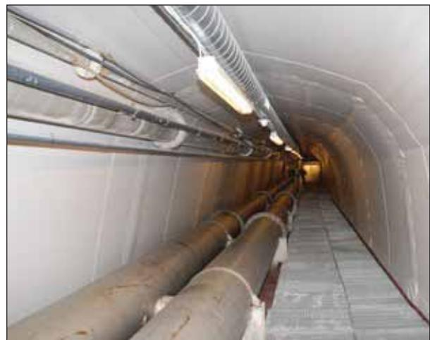
Figures 1 and 2: The picture to the left shows a typical situation in a pipe access tunnel where you have a wet and humid environment that gives corrosion problems to steel pipes and electrical equipment. To the right we see a picture of a complete different result after the installation of WGTS. The humidity is now under control and the lift time for the assets has increased dramatically.
