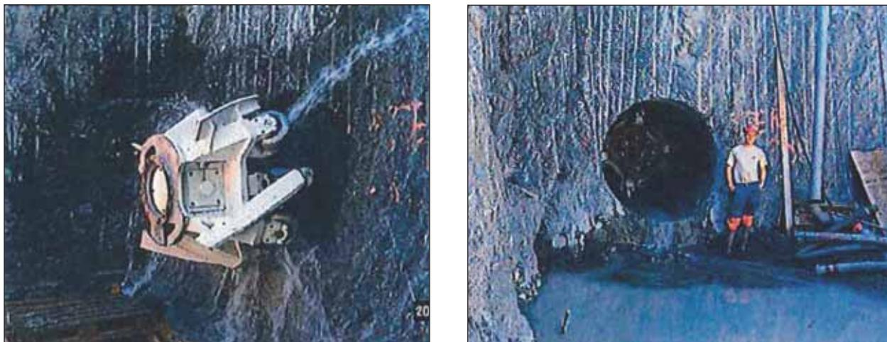
Figure 4 - Hesthaugen, Sandvika. Horizontal small tunnel,  $\phi$  1850 mm, length 295 m, inclination = 0,07 % for leading surface/waste water away from the railway lines.
