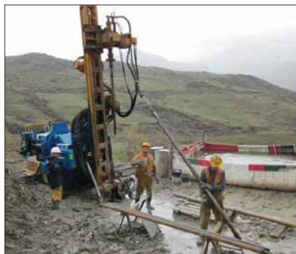
Figure 5: Core drilling in the Flysch
