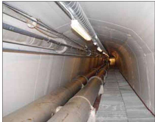
Figures 1 and 2: The picture to the left shows a typical situation in a pipe access tunnel where you have a wet and humid environment that gives corrosion problems to steel pipes and electrical equipment. To the right we see a picture of a complete different result after the installation of WGTS. The humidity is now under control and the life time for the assets has increased dramatically.
