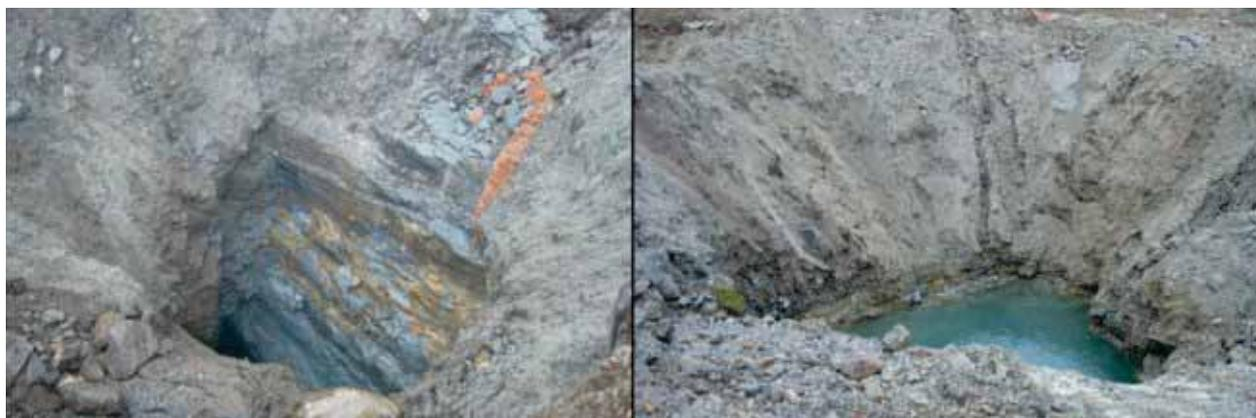
Fig. 2 - Sinkhole nearby Stutakvelven intake gate house in fully drained (a) and fully water filled (b) conditions (Courtesy: Norsk Hydro).
