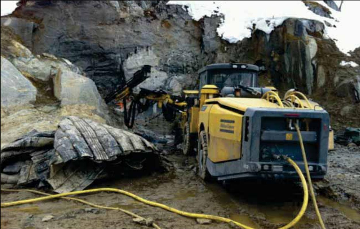
Figure 8 Securing and spiling
