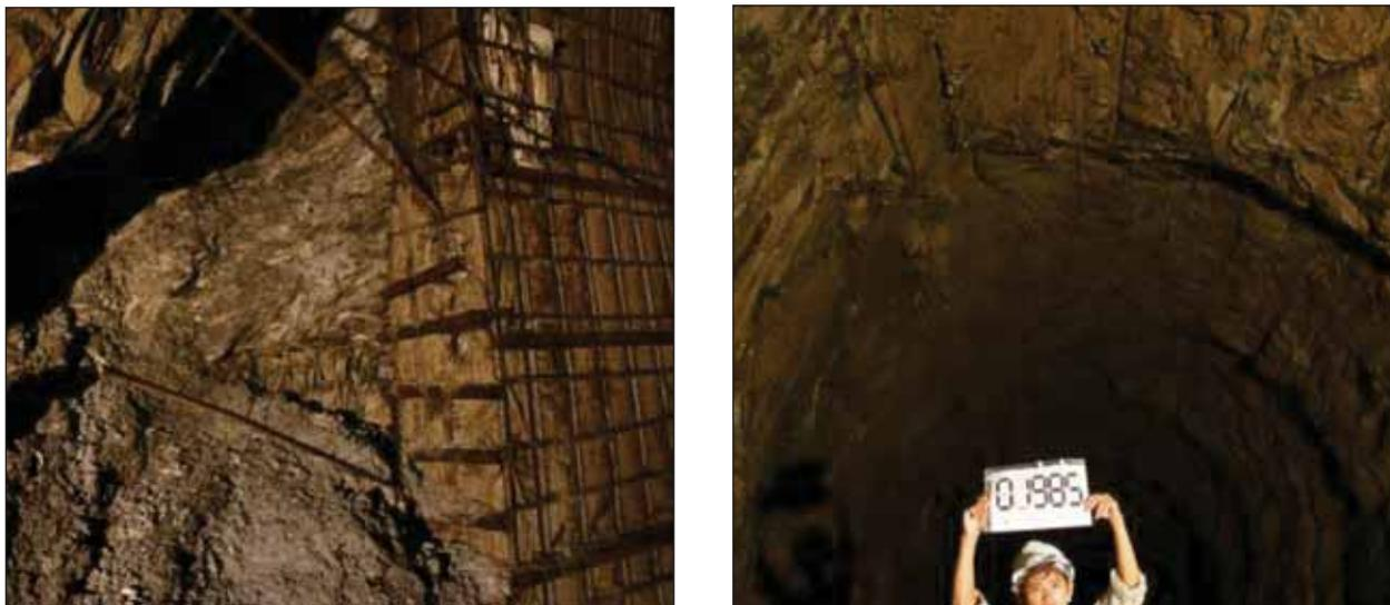
Figure 4 - Typical “Extremely Poor” (left hand side) and “Fair” (right hand side) rock mass conditions.
