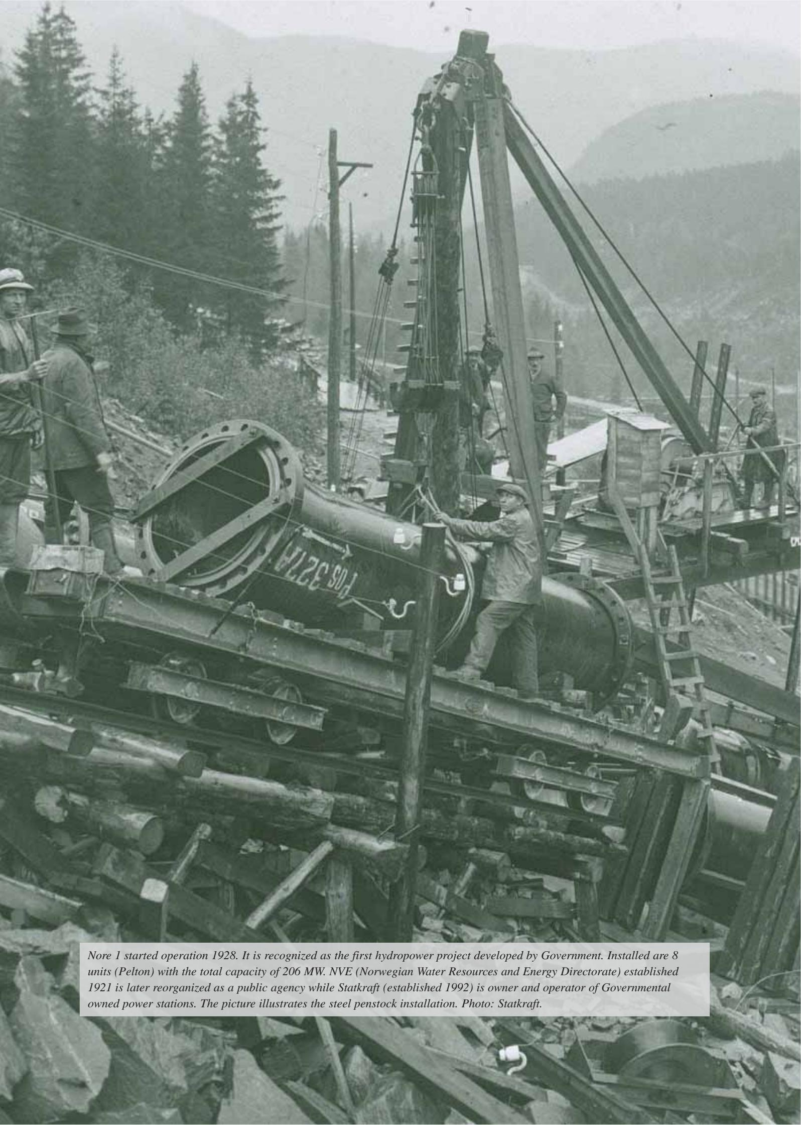
*Nore 1 started operation 1928. It is recognized as the first hydropower project developed by Government. Installed are 8 units (Pelton) with the total capacity of 206 MW. NVE (Norwegian Water Resources and Energy Directorate) established 1921 is later reorganized as a public agency while Statkraft (established 1992) is owner and operator of Governmental owned power stations. The picture illustrates the steel penstock installation. Photo: Statkraft.*
