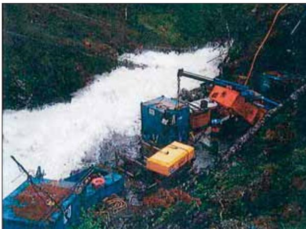
Figure 3 - Gryto Hydropowerplant, Hardanger, Length = 500 m. Diameter  $\phi$  770 mm, inclination 45°.
