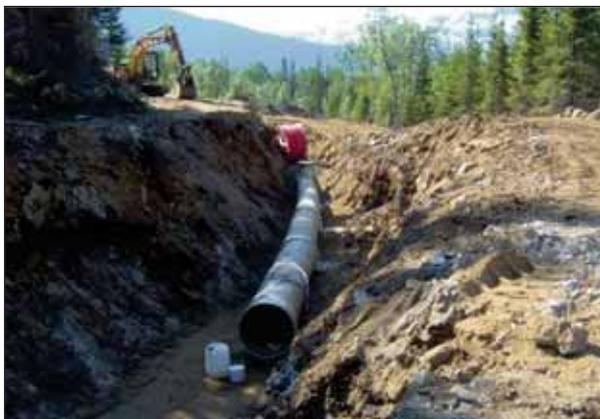
Figure 1. Installation of penstock in ditch
