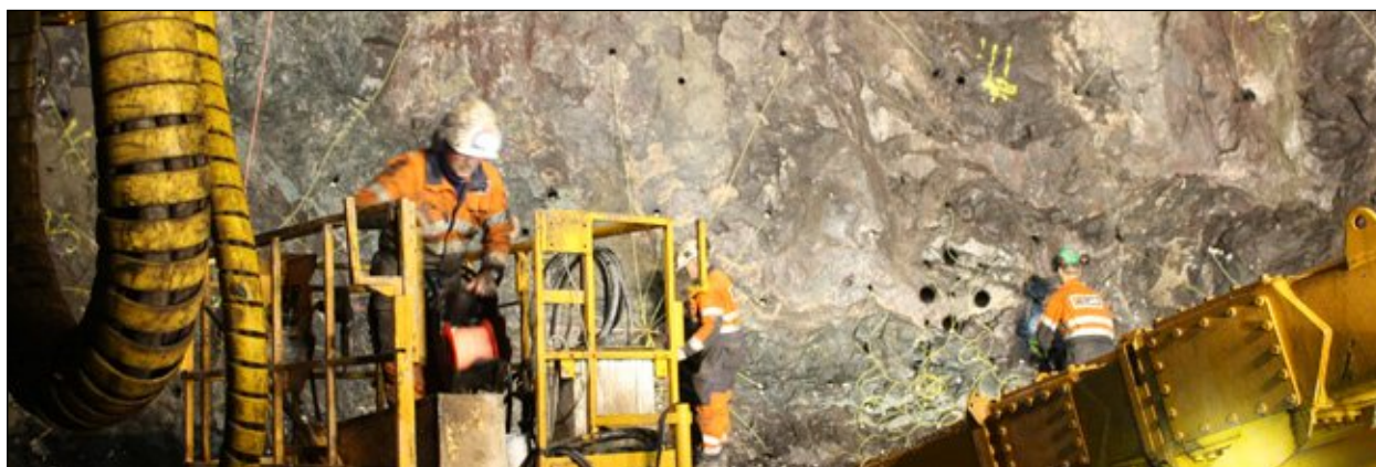
The crew at face. Charging of another round is finished. Photo Ruth Haug, LNS.
