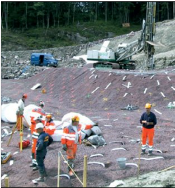
Figure 2 Veidekke solution with vertical drainage combined with temporary rock fill.
