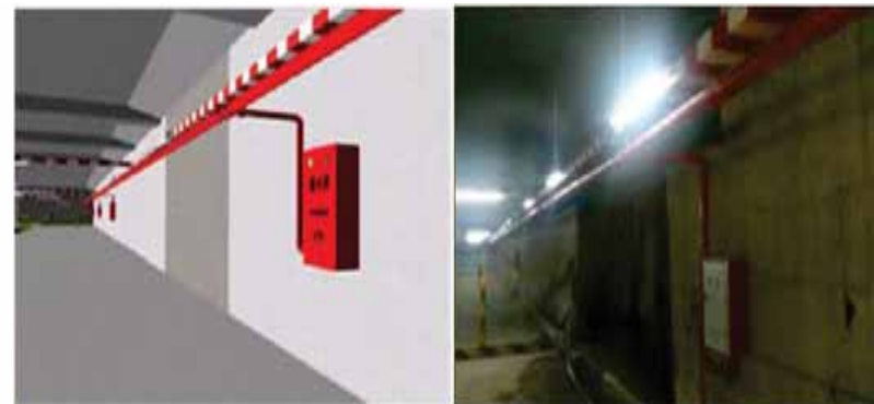
Figure 8 A screenshot of the 3D model related to an order sheet for the installation of a fire box and a photo on site after the work was completed
